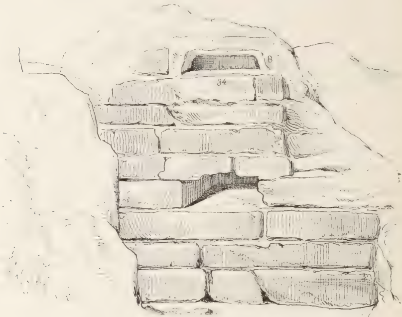
FIG. 41.—Wall of crude brick.
